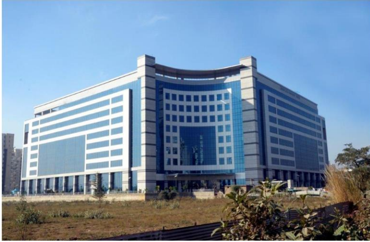
BESTECH BUSINESS TOWER SOHNA ROAD
